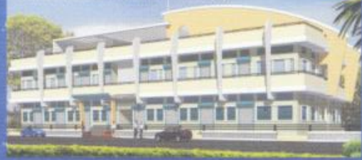
Unico Industrial Park - Vasai (E)
